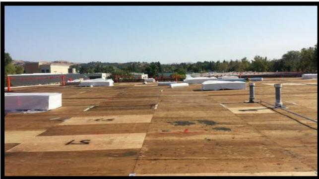
*Where needed, new roofing plywood has been installed. Structural inspections have been completed.*
