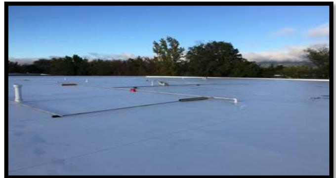
*The new roof has been installed. HVAC equipment "curbs" will be installed on which the new air conditioning units will be mounted.*
