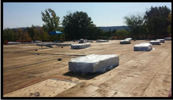
Demolition on the roof is now complete. Structural inspections have been completed. The new roofing material is now loaded.
