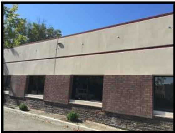
Blueline Construction is now completing all seismic upgrades to the building. The bolts you see on the exterior are part of the new structural system.
